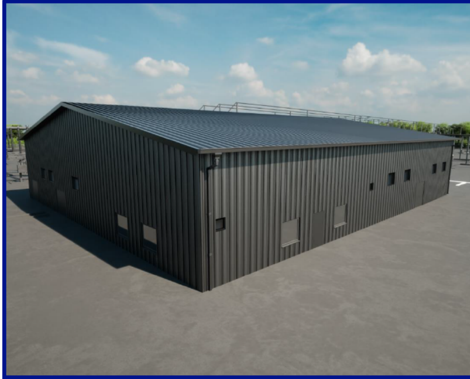
Figure 37: Monk Fryston Control Building Finish - Grey Cladding
