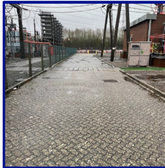
Figure 32: Block Paving (Source: MM Site Visit)
