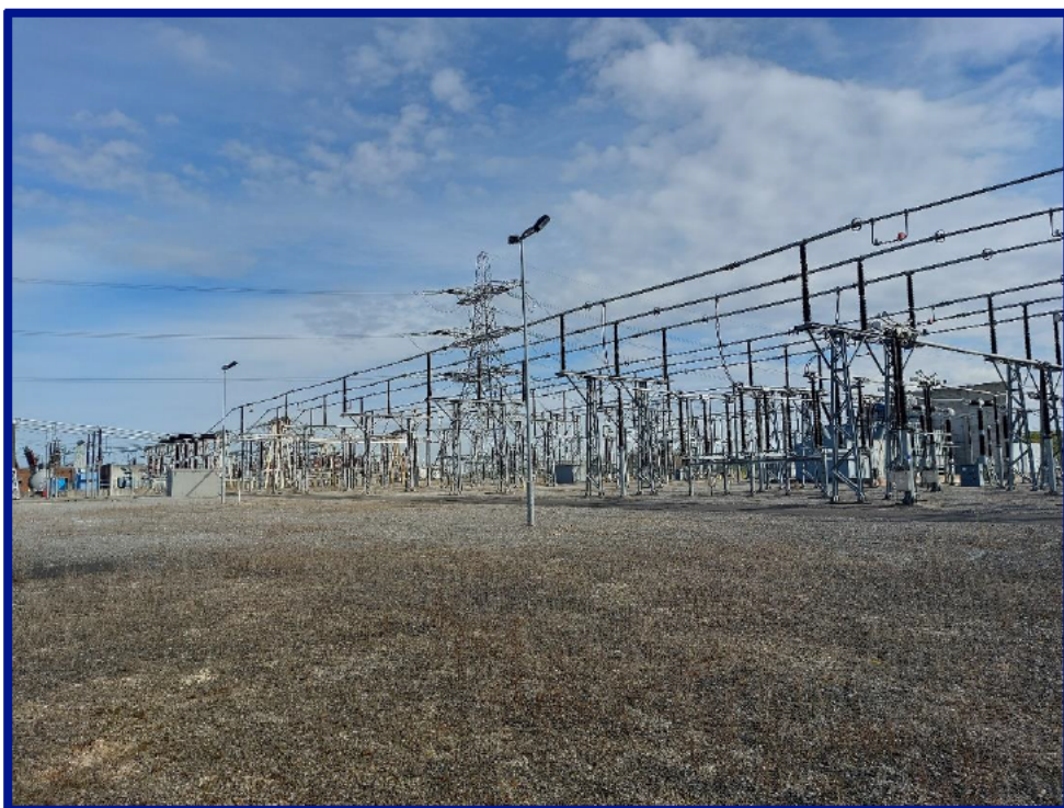
Figure 2: Existing Substation - Monk Fyston (Source: MM Site Visit)
