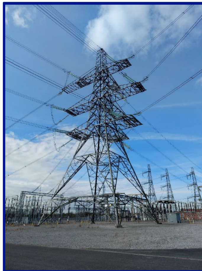
Figure 3: Existing Substation - Monk Fyston (Source: MM Site Visit)
