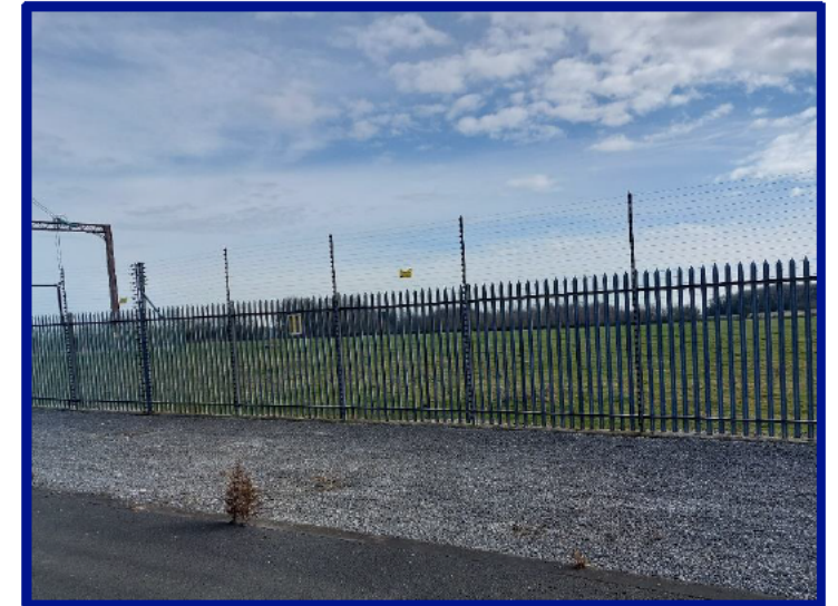
Figure 30: Security Fence (Source: MMD Site Visit)
