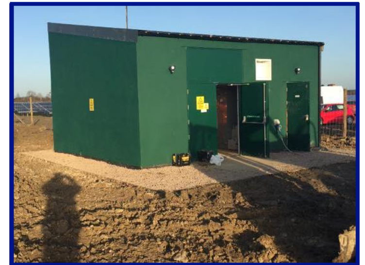
Figure 34: Green DNO Building (Source: Integral Utility Services)
