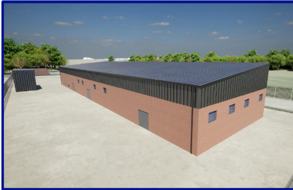
Figure 25: Overton Control Building Finish - Cladding and Red Brick
